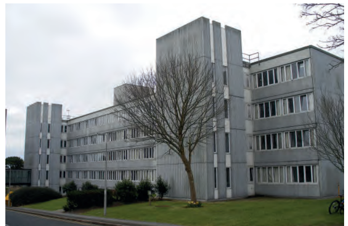
Large panel block (c1965). These make up less than 1% of the UK housing stock.
