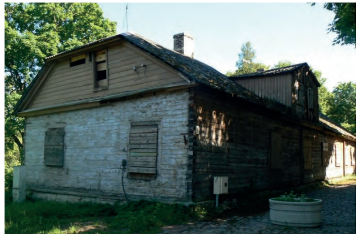
Vacant dwelling in popular village, awaiting refurbishment
