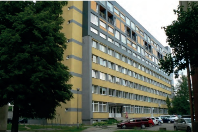
Pre-fabricated concrete block of flats in Vilnius, originally built around 1965 and refurbished through a municipal scheme. Works include insulated over-cladding, double glazed windows and improved district heating.
