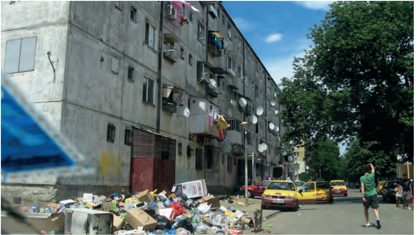
Small concrete panel construction flats, Romania
