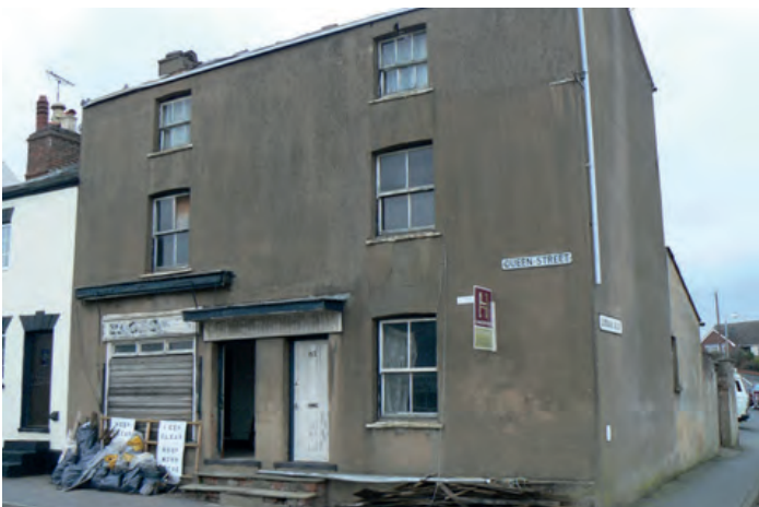
Cold, damp and rot in c1850 end terrace house
